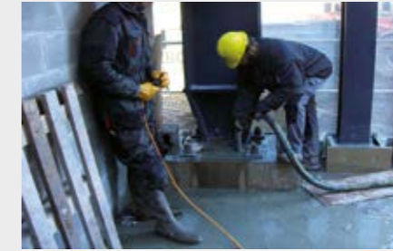
Filling steel columns
