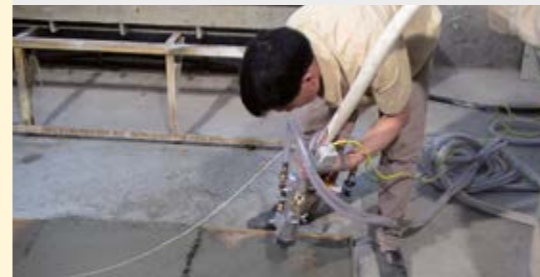
Making fibre-reinforced concrete slabs
