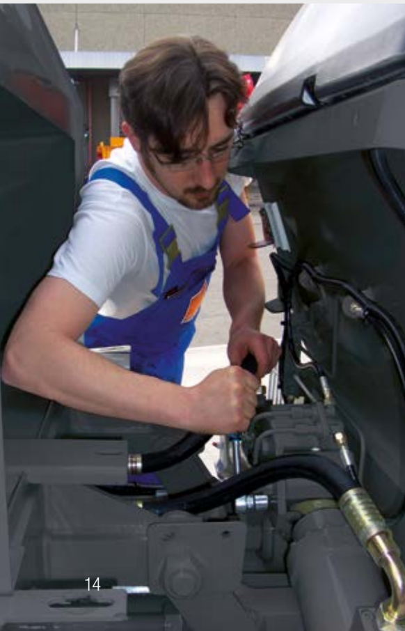
Good access for service work
