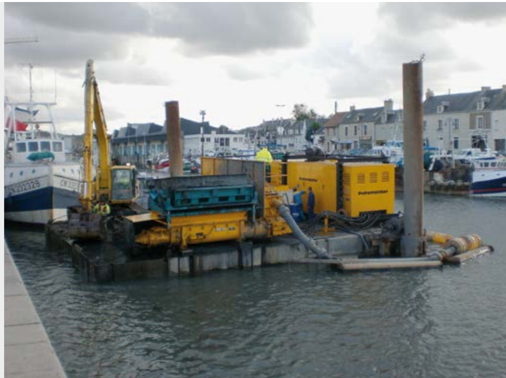
Sludge handling system operating in a canal in France with an S-tube pump and diesel-driven power pack mounted on a ponton
