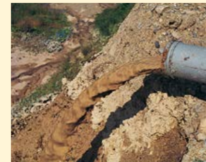
Removing slurry from a tunnel
