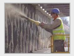
Fine concrete pumps like the P 715 are among the most versatile systems. You can use them for shotcrete or for pumping fine concrete of up to 16 mm.
